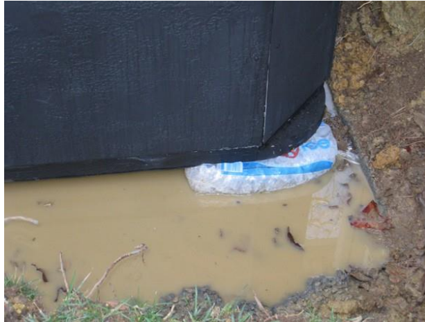
Figure 8. Swim Spa And Exercise Pool Position in Excavation on Ice Bag
