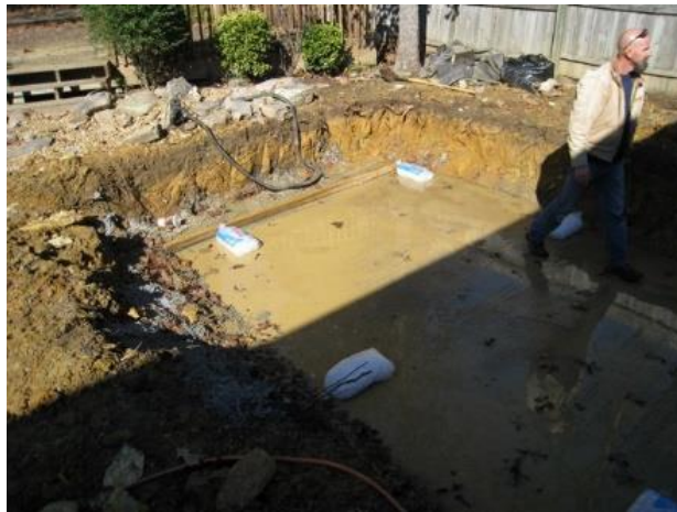
Figure 7. Ice Bag Positioning in Excavation
