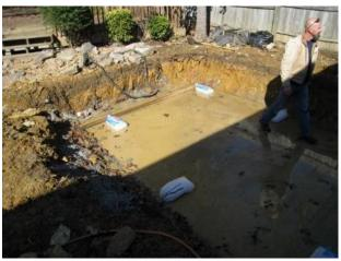
Figure 7. Ice Bag Positioning in Excavation Crane the spa into position like a normal spa delivery.
